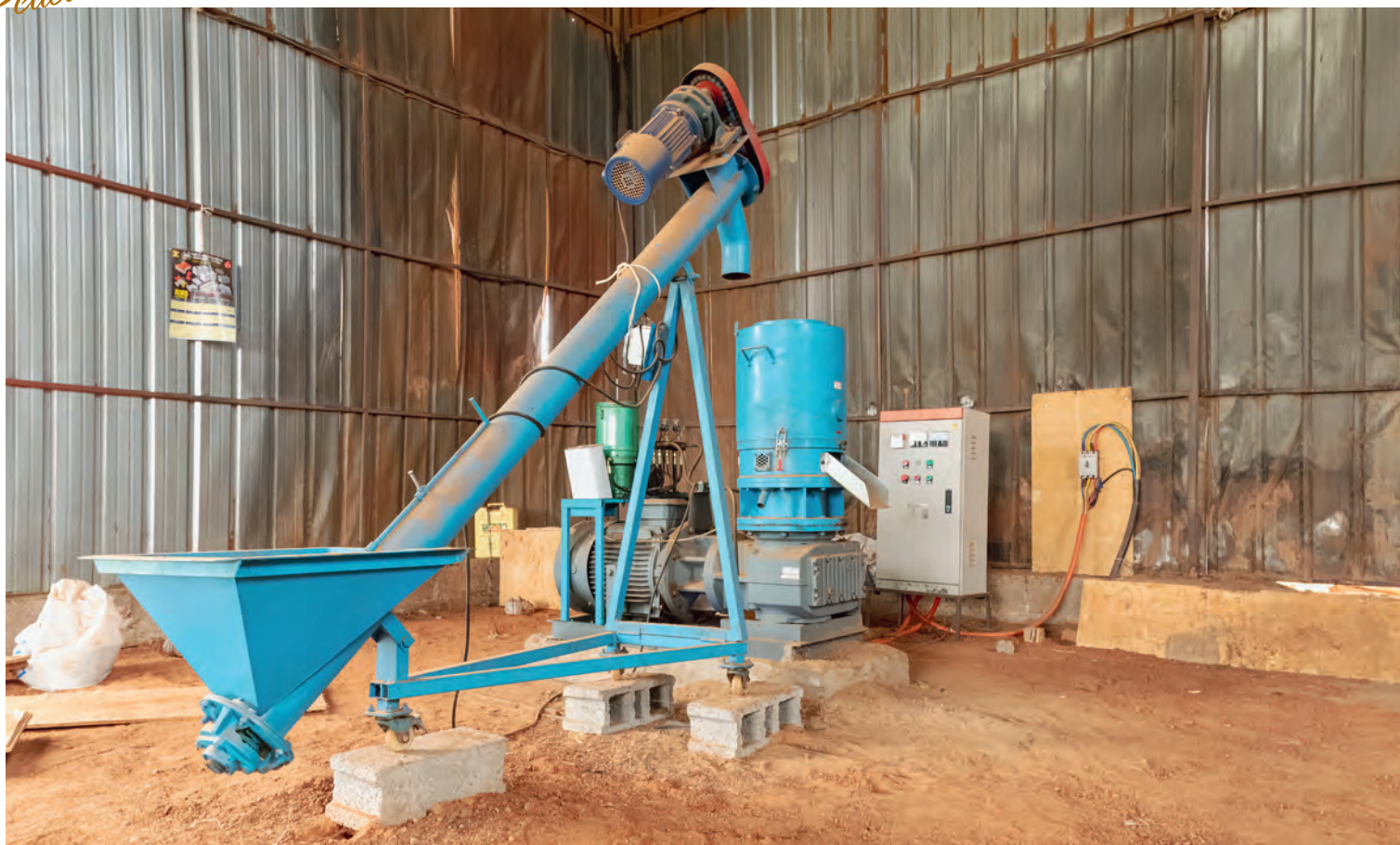
A biomass pelleting unit installation in progress for Tru Biomass at a site on the outskirts of Kampala.
