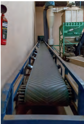
(Above left) The counter-flow sieve cooler. (Above right) The bagging station conveyor that brings the bagged pellets into an adjoining warehouse with the pellet cooler in the background.
