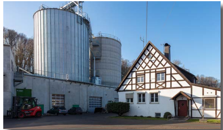
Towering behind the Bullinger home office, the "Bulli Pellets" plant footprint comprises the two silos, with the plant housed below the concrete silo on the right, and bulk truck loading bay located at the rear of the lefthand silo.
